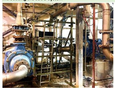
The LOBO System is a versatile work platform product that combines the flexibility and strength of traditional scaffolding with the simplicity and mobility of tower systems. The unique and patented hand adjustable clamp, when combined with the tube, allows the technician to create a work platform, of any shape or size, without the need for any tools.
